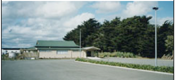
Large Septic and Peak Load Storage Tank situated behind hall.
