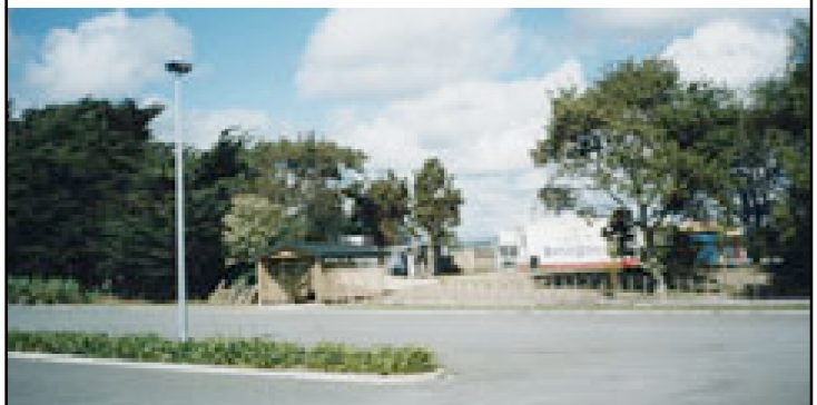
Filtered Effluent Timer Dosed into LPED Trenches in narrow garden areas after crowds have gone home. Ideal for Marae's etc.
