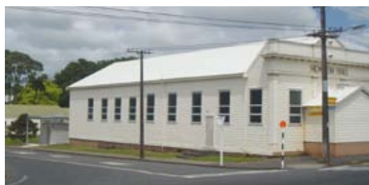
Okato community hall with public toilet down side street.
