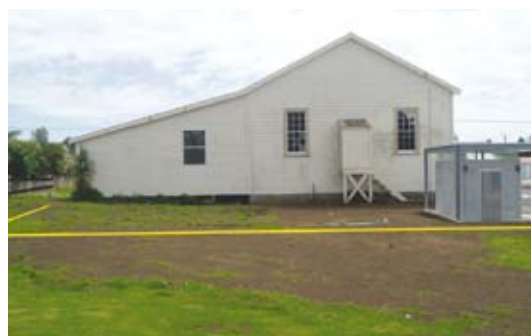
Okato Community Hall and public toilet. The only land available for effluent disposal is the narrow strip immediately behind the hall and to the left of the public toilet – approx 100m 2 .
