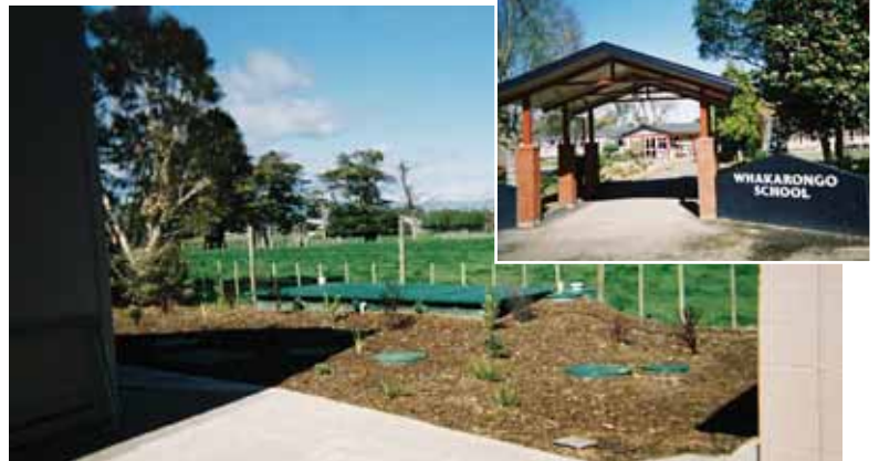
The Treatment Plant.
