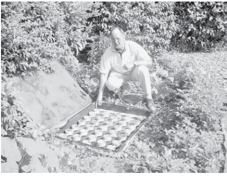
Figure 4. Dave Miller inspects a fabric recirculating packed bed reactor located close to the residence. Treated water of BOD 5 /TSS of less than 5/5 ppm safely irrigates the garden.
