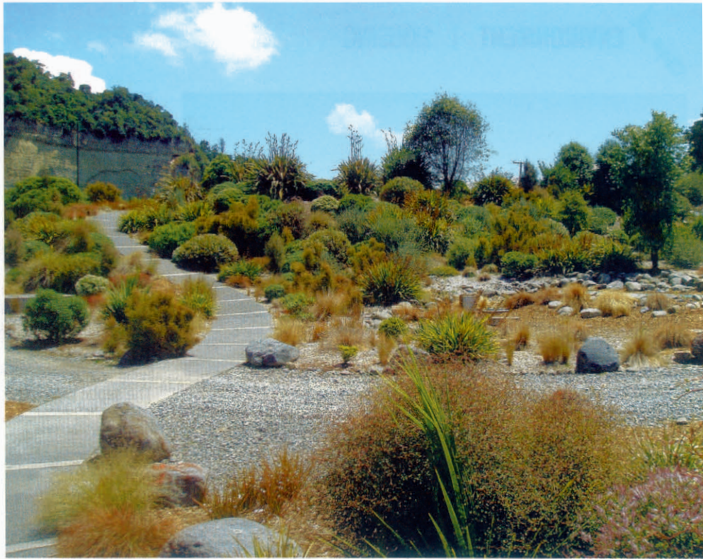
Secondary treatment system with attractively planted garden hiding the drip lines.
