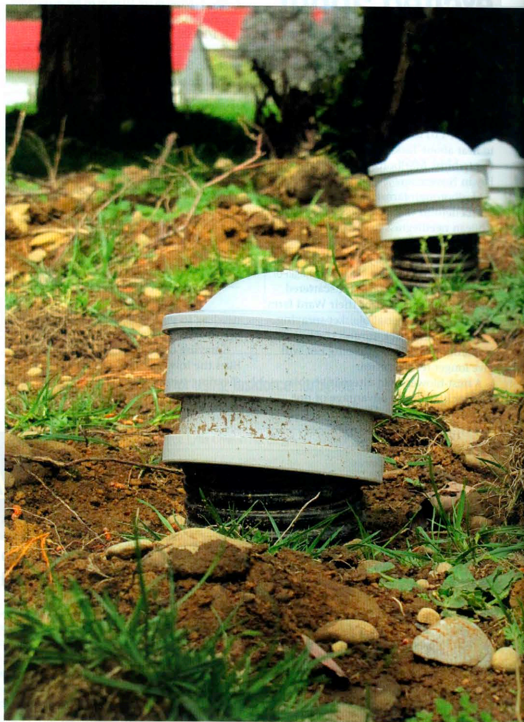
The mushrooms at the end of low-pressure effluent dosing trenches, a cheaper option on the right soil type.
